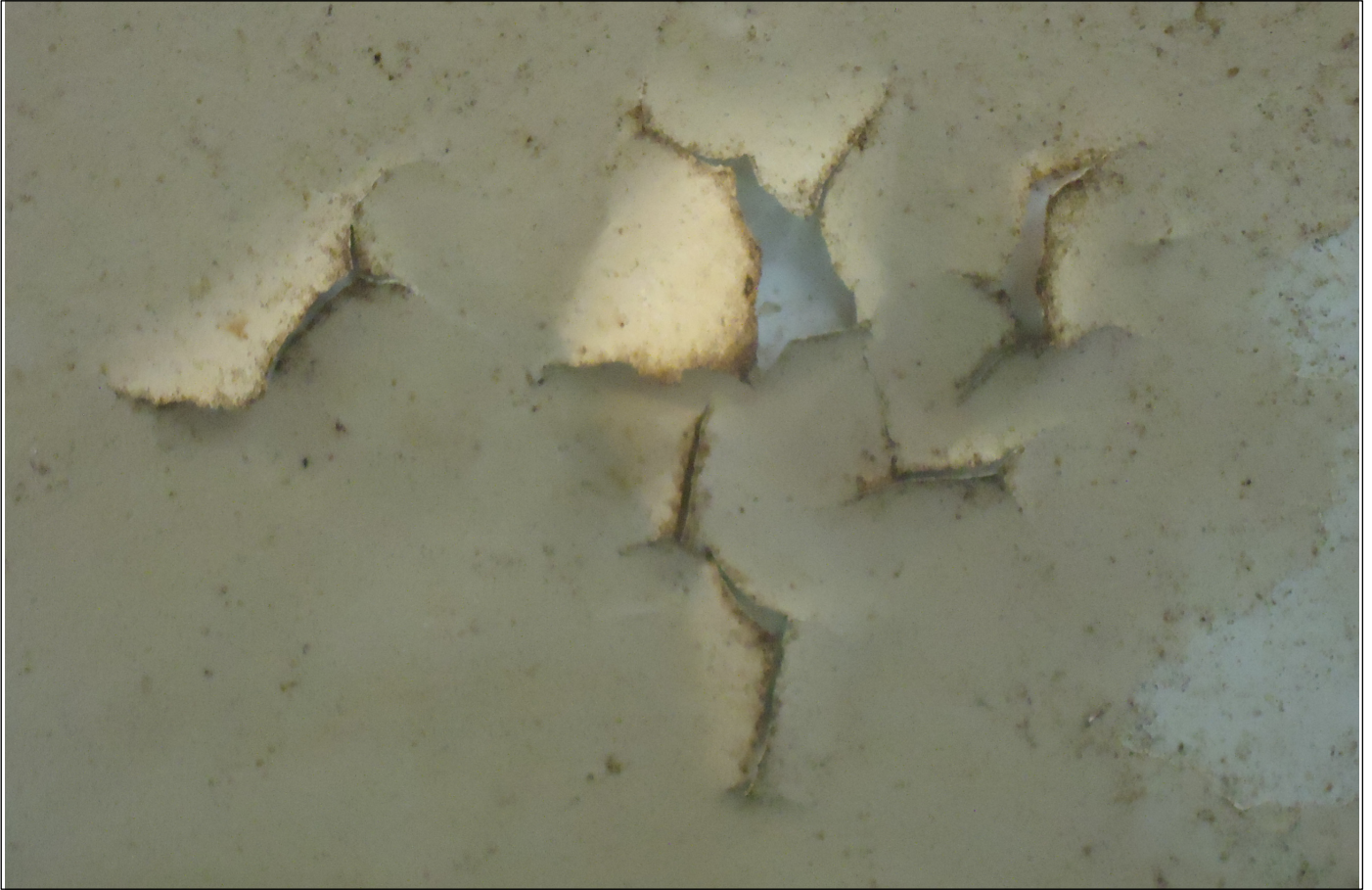
6.1 Kitchen/Dining. The ceiling.
